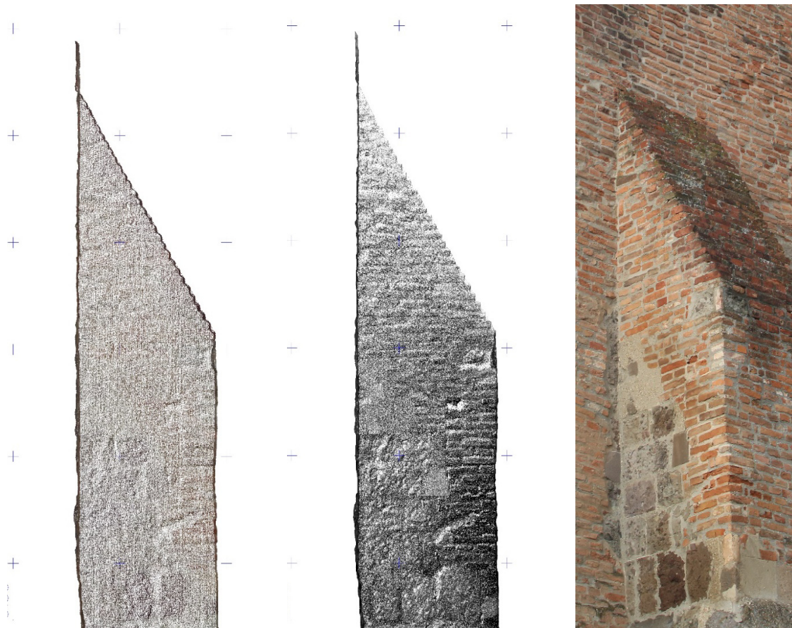
Figure 7. True colored (left), intensity colored (middle) point cloud and a photo (right) of the same wall part
