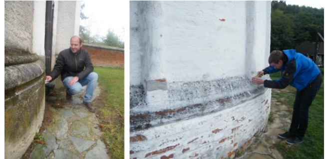
Figure 6. Good examples to right identify ground wall points at Ják (rough walling) and Kallósd (brick walling) church
