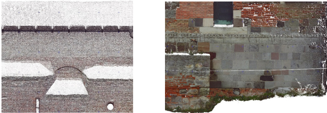
Figure 6. Merged (TLS + UAS) point cloud on orthoviews about a higher wall part and roof (left) and bottom of a wall (right) outside
