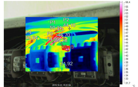
Fig. 8. Overloaded wires
