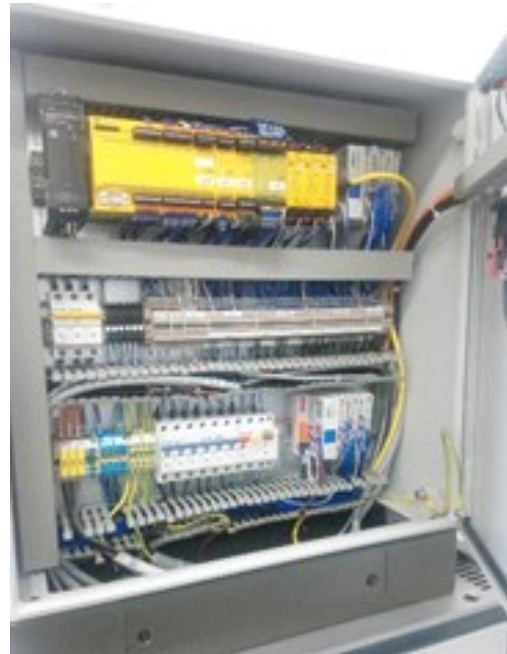
Fig. 9: Electrical cabinet of the safety PLC
