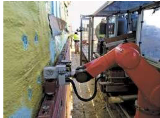
3. Figure Construction Robotics' SAM 100 in service
