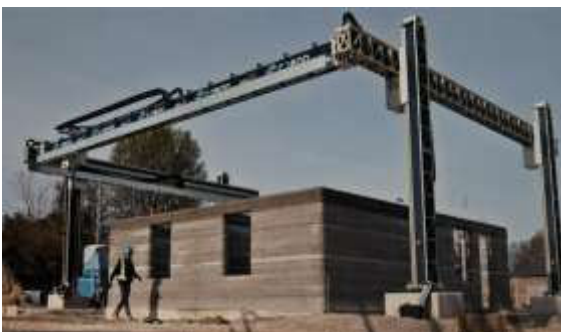
2. Figure 3D printed house by COBOD
