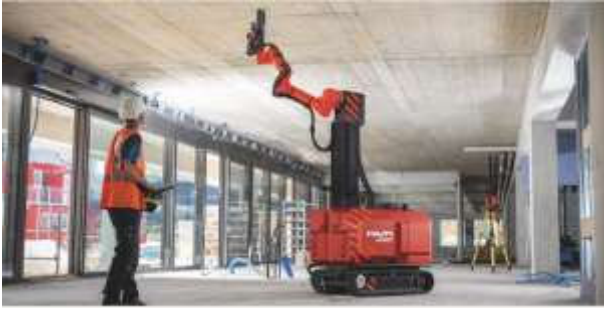
8. Figure HILTI Jaibot drilling mobile robot in operation [14]
